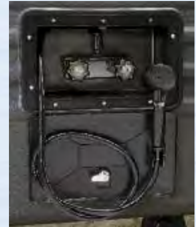
Hot and cold outside shower reduces tracking dirt indoors
