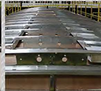
Walkable steel truss roof system
