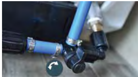
Water heater bypass & winterizing valves make draining the system for winter storage a breeze.
