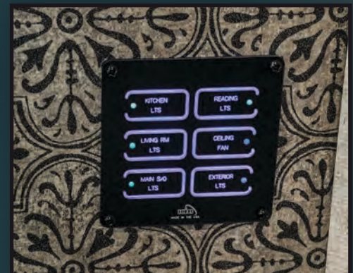
MULTIPLEX LIGHTING SYSTEM
