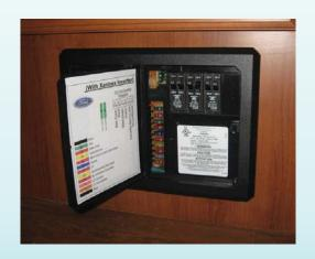
The converter is equipped with an automatic switchover relay to prevent both the generator and the external power cord from being connected to the converter at the same time. When either the external power cord or the generator is being used, both the 110 volt AC system and the 12 volt DC system will be activated inside the motorhome. When neither of these is connected, the 12 volt auxiliary batteries will activate only the 12 volt DC system.
