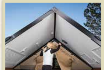
SET UP THE SIDEWALLS
