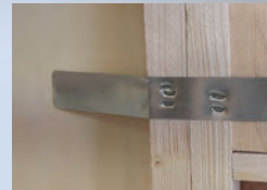
Hurricane Straps Add Strength and Safety
