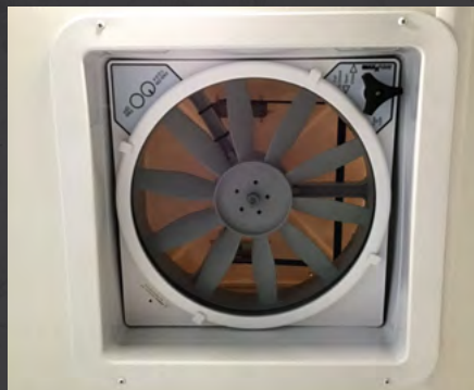
High Output Attic Fan in Bathroom
