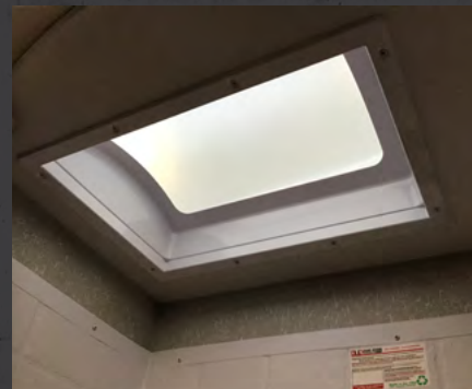
Skylight over Shower
