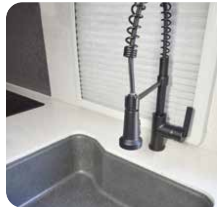
Residential faucet fixtures.
