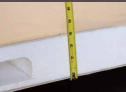
4" thick roof with built in insulated A/C ducts
