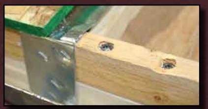
Unlike our competitors whose roof rafters are simply stapled, North Country's roof rafters are screwed securely to the sidewalls, meaning no worries about the structural integrity and solidity of North Country's roof system!
