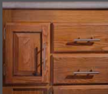
Upgraded Cabinetry Hardware
