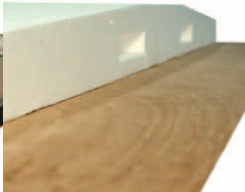
Radius roof foam with built in insulated A/C ducts
